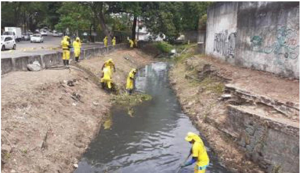
Figura 11: Limpeza manual executada no canal do Parnamirim
